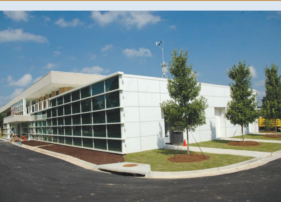
The 4,500 ft 2 learning center has a total seating capacity of about 400 when three main meeting rooms are used in conference seating configuration. The three rooms can also be subdivided to create seven individual meeting rooms.
