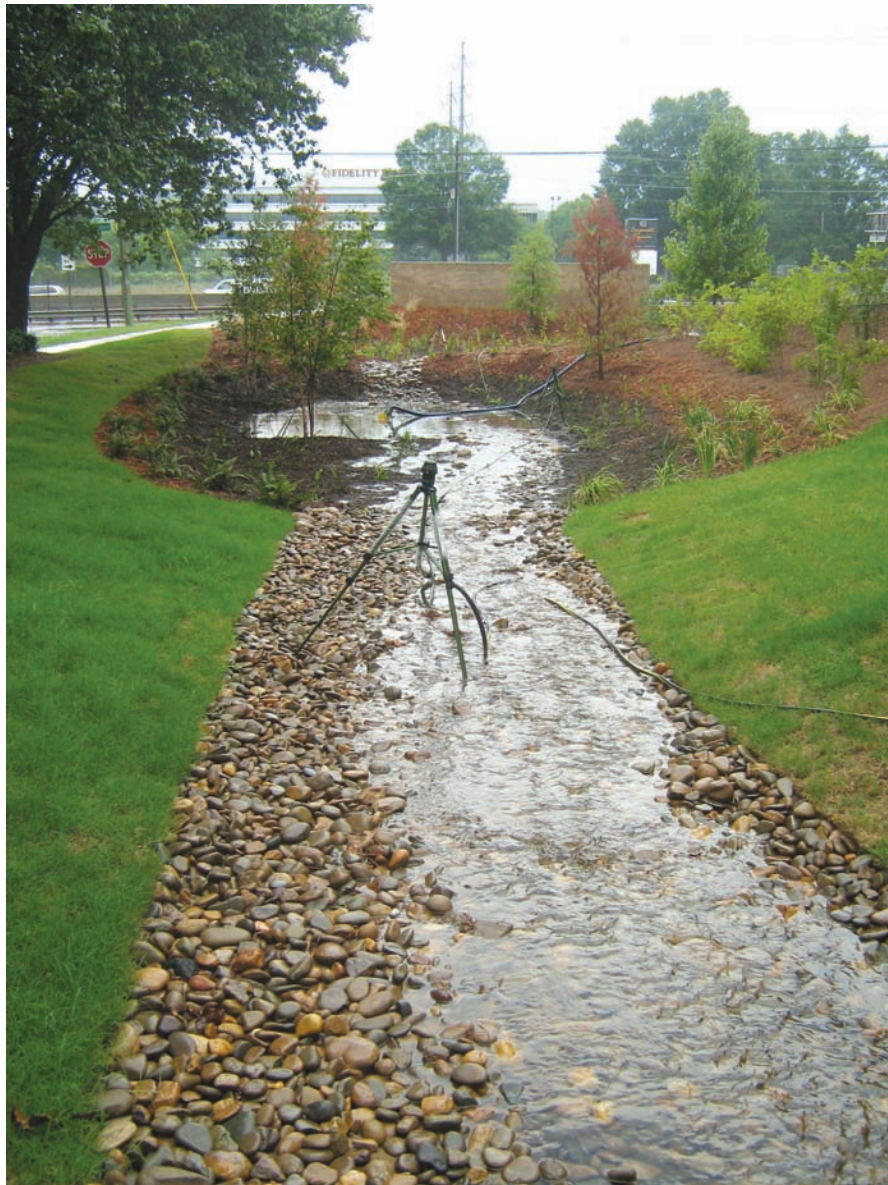
ASHRAE has reduced the amount of site runoff by 34% and reduced the runoff rate by 30% by implementing a storm water detention and bioretention system.
